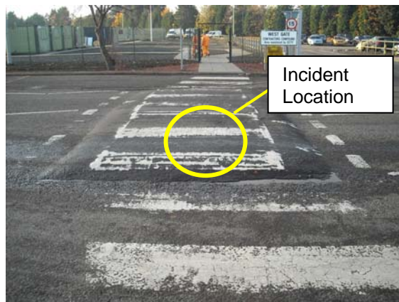
Figure 1 - Road Crossing at Site Gate Entrance
